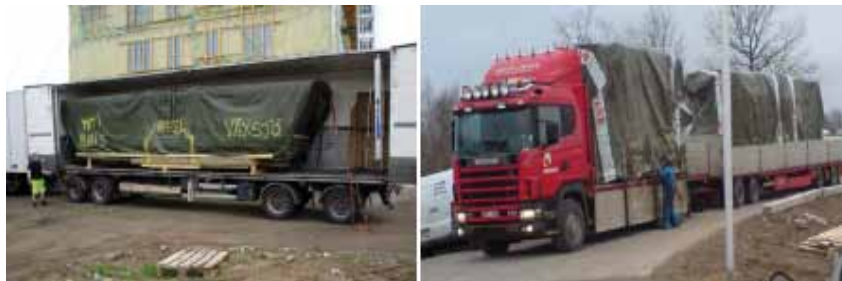
Transport of wall and floor elements at Limnologen [14]
